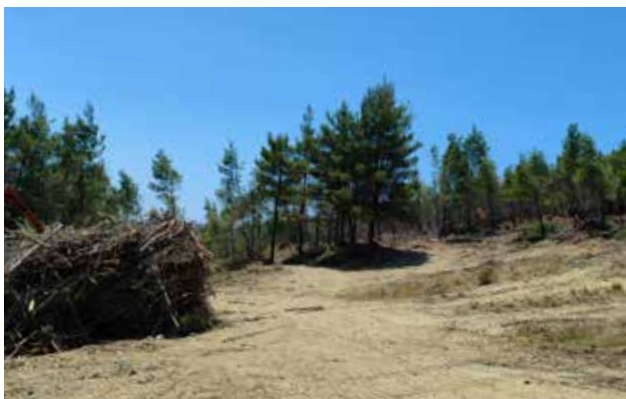
Creation of firebreaks in Attica, Greece. Photo courtesy of ILVERDE.
