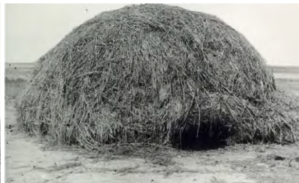
Illustration 3: Finished construction using native grass to insulate
