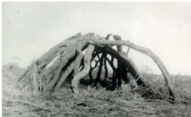
Illustration 2: Traditional shelter under construction
